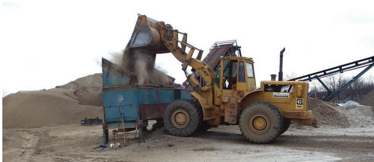
Van Geiger dumps a load of 304s into the screen plant where it is screened into 310s, 57s, and 4s.
